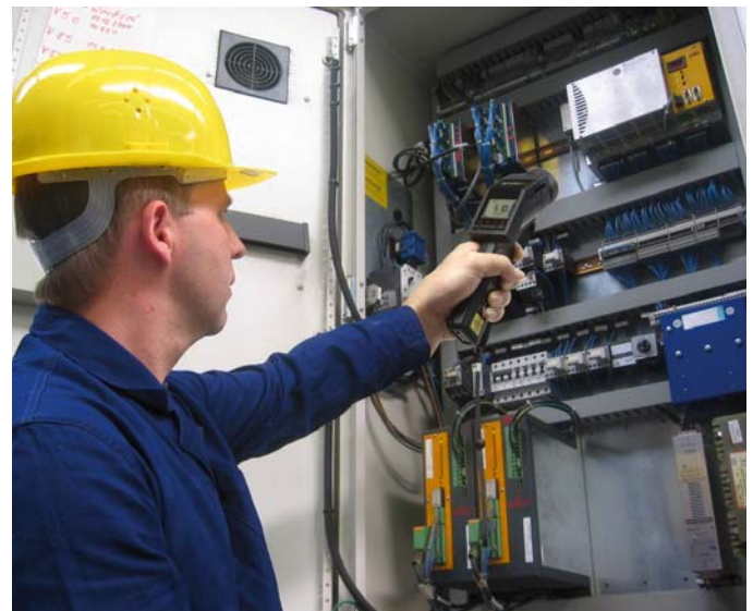
Picture 1: Temperature measurements on stressed components in a switch cabinet using the optris LaserSight LS
